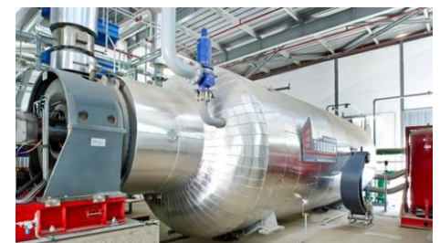
Waste Heat Power Generation (ORC)
