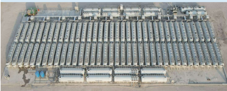
Construction Camp (IRAQ) 3600KL/Day
