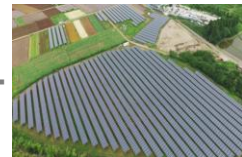
Solar power generation
