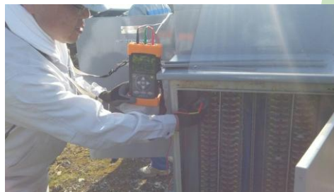
Sumba field inspection (2017)
