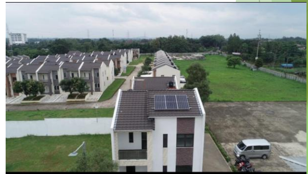
Residential Development in Depok
