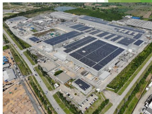
Solar power generation (example in Thailand)
