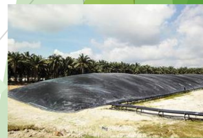
Bio Gas Power Generation
