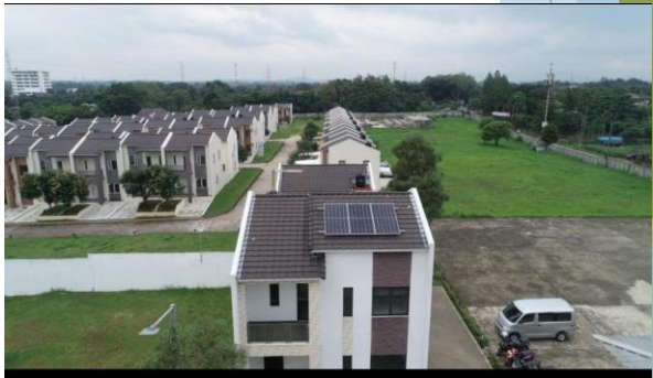
Residential Development in Depok
