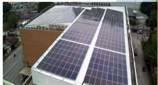
(Solar Power Plant)
