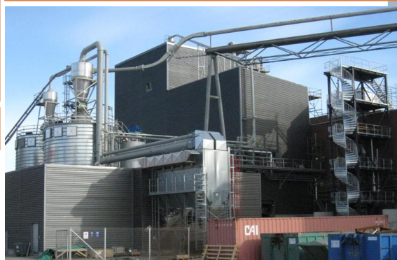
Location: Varkaus, Finland Customer: Stora Enso Oyj & Neste Oil Corporation Start-Up Year: 2009 Capacity: 12 MWth Scope: Biomass Gasifier Fuel: Biomass, Forestry Residues Gasifier Type: CFB
