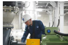
On-site Pump Assessment
