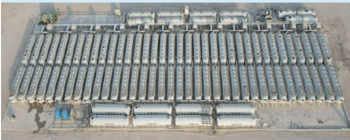
Construction Camp (IRAQ) 3600KL/Day
