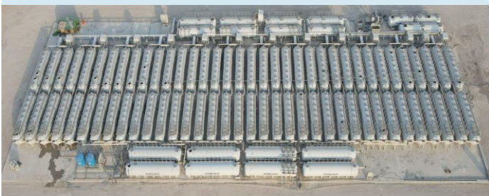
Construction Camp (IRAQ) 3600KL/Day
