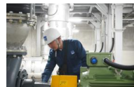
On-site Pump Assessment
