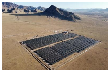
Tenaga Surya + BESS
