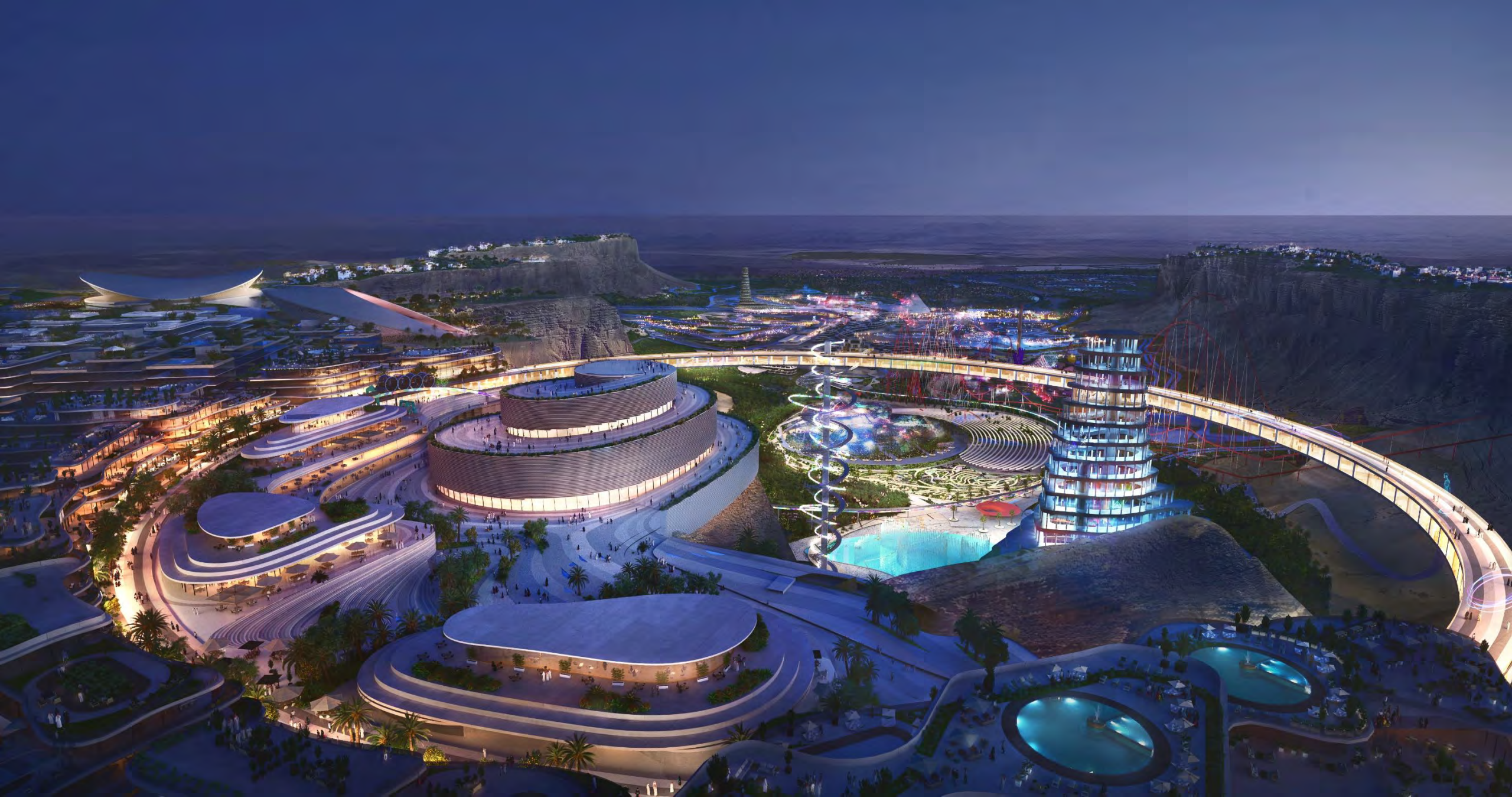
Aerial view of the Performing Arts Center and the cliff side plaza
