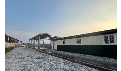
Tempat Pengolahan Sampah Terpadu (TPST) Integrated Waste Processing Facility
