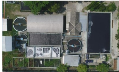
IPAL Waste Water Treatment Plan
