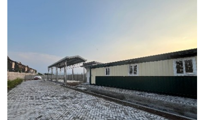
TPST Integrated Waste Processing Facility
