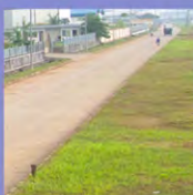
cast concrete street jalan cor beton
