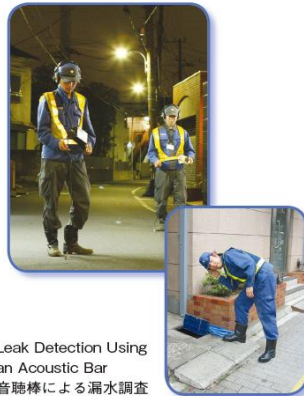
Leak Detection Work at Night 夜間の漏水調査作業
