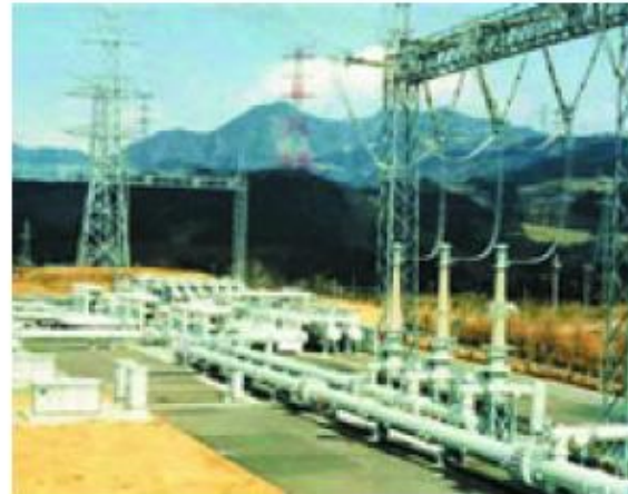
Gas Insulated Switchgear
