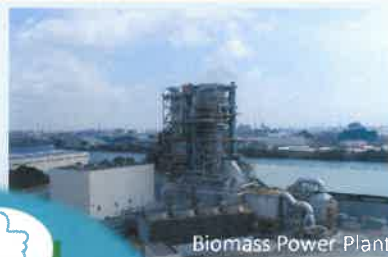
Biomass Power Plant
