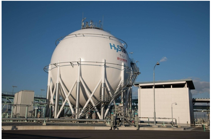
A hydrogen storage tank and loading system at a liquefied hydrogen receiving terminal in Kobe © Bloomberg
