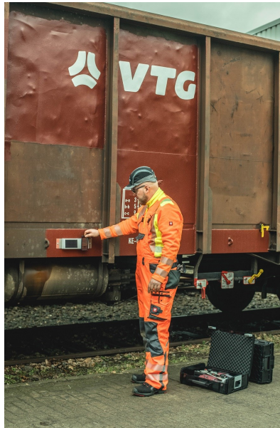
Installation of a Nexiot device
