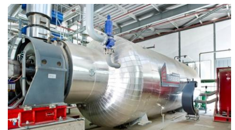
Waste Heat Power Generation (ORC)
