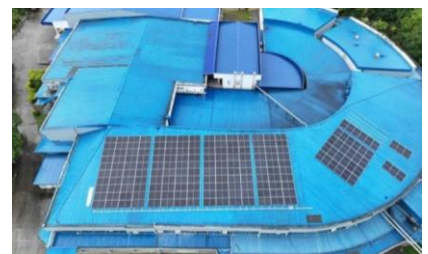
Client: AM-Europharma Capacity: 115.2 kWp
