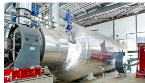
Waste Heat Power Generation (ORC)
