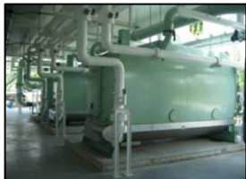
Exhaust Heat Recovery System
