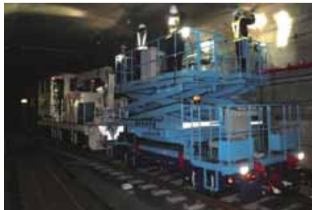
Carrying out sophisticated maintenance
