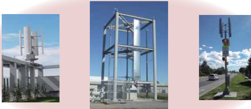
Wind turbine generators
