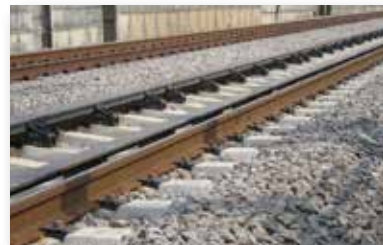
Derailment prevention guards , unique and effective countermeasures against earthquake disasters in Japan
