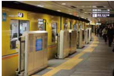
Large-scale renovation underway for the entire Ginza Line, the oldest subway line in the Orient
