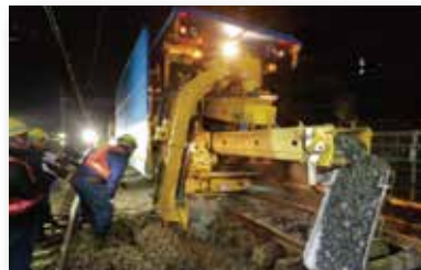
Maintenance work during the night hour , an essential element for safe and reliable operation
