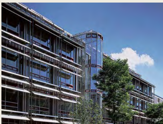
The headquarters of HAWE Hydraulik SE in Germany.
