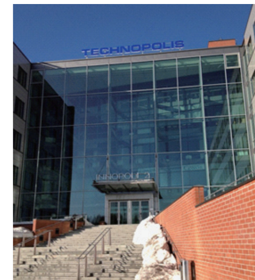
Office Yui's premises in Espoo City, Finland
