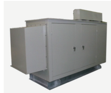
Uninterruptible Power System (UPS)
