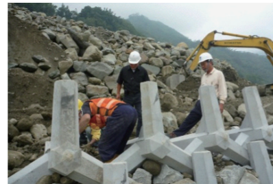
Construction method using branch-shaped concrete blocks
