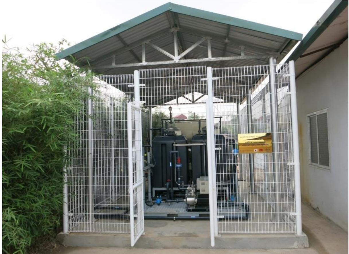
Process: Chlorination → Rapid SF → AC → UF (20m<sup>3</sup>/D)
