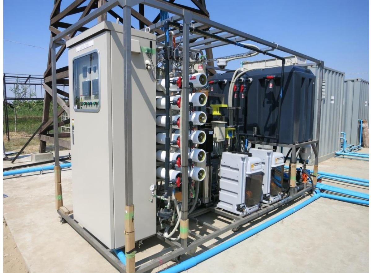
Process: Submerged UF → RO membrane (Pilot)
