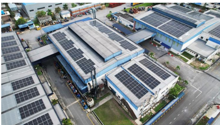
Solar PPA of 1,097 kWp for Toyochem Specialty Chemical Co.
