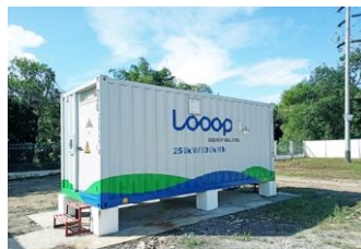
Container-type battery storage system
