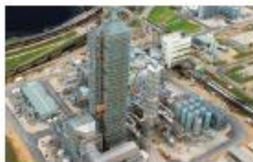
World's Largest CO2 capture plant (America, Petra Nova)
