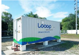
Container-type battery storage system
