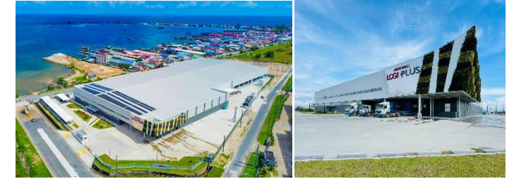
AEONMALL CAMBODIA Sihanoukville FTZ Logistics Center
